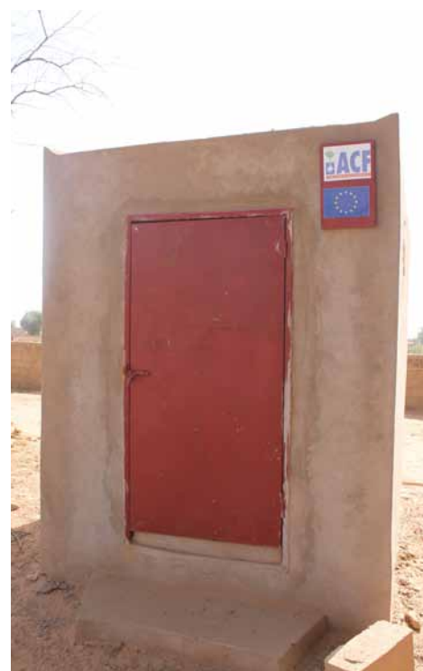
Picture 6: Stock for medical waste built in a health care facility which does not have an incinerator
